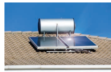
Installation on a sloping roof
